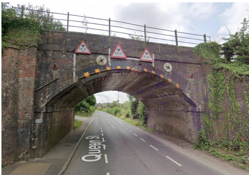
Figure 6-2: Wilton Road Bridge
