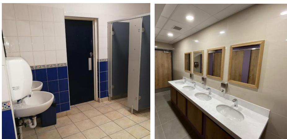
Figure 7-17: Before and after images of improvements to York Lorry Park
